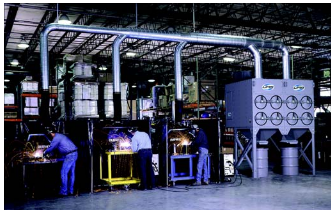
Figure 3. Downward flow cartridge weld fume dust collector with source capture.
