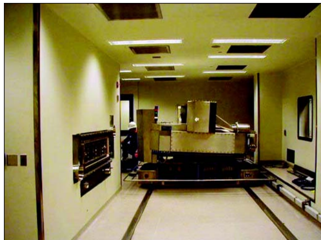
Figure 6. Transfer cart with barrier isolator.
